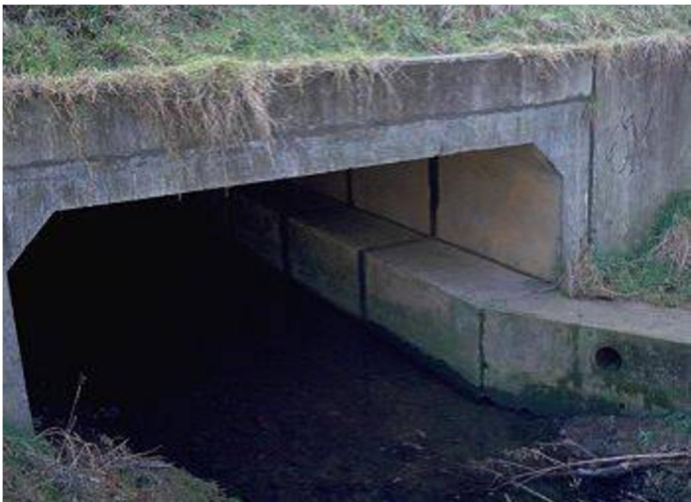
Box culvert modified with ledge for small animal passage (Jackson, 2004)
