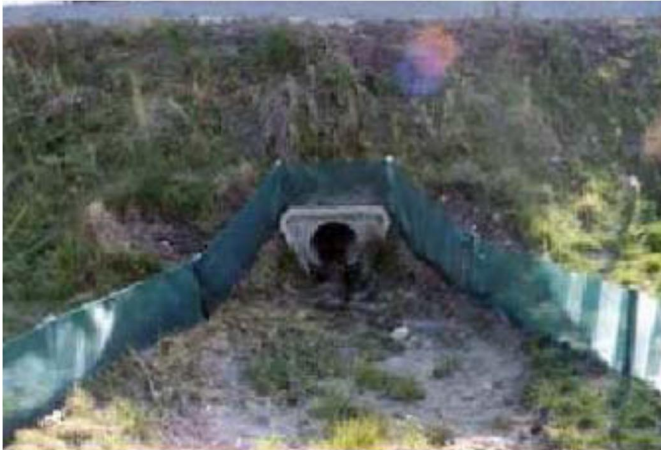
Small pipe culvert with mesh fence for small mammals and amphibians (FHWA/US DOT, 2002)
