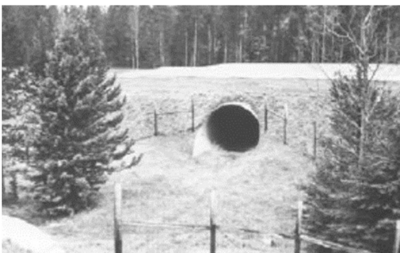
Pipe culvert with fencing for medium mammals (NCHRP)
